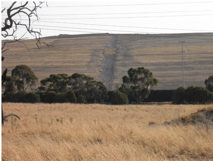
Fig. 4. An engineered channel on a post-mining landscape.
