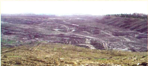
June 4, 2004 – After the material was placed by precision GPS-guided dumping, dozers equipped with Leica's Dozer 2000 knocked off the edges of the lifts and completed shaping of the complex slopes and valley bottom channels.
