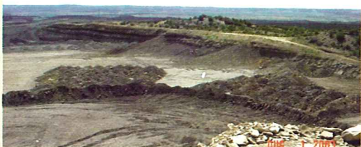
August 1, 2003 – As precision GPS-guided dumping continues, the general shape of the GeoFluvTM-designed landform begins to emerge. Valleys will be cut between the fill against the highwall and the cut material will supplement the ridges.
