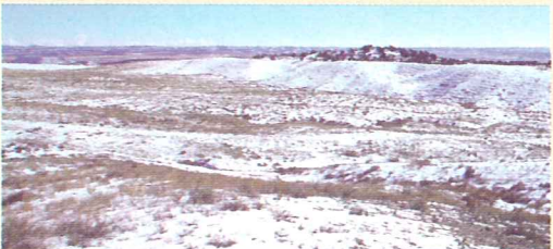
December 13, 2005 – A half-year after plants began to sprout and the stable and functional GeoFluvTM-designed landform already harmonizes with the surrounding landforms. The highwall is gone, replaced by a stable and functional north-facing special landscape enhancement feature that will promote tree growth. This feature, about 1,200 feet (366 m) long, enhances the post-mining land use and eliminated the need to move huge volumes of material against the former highwall.
