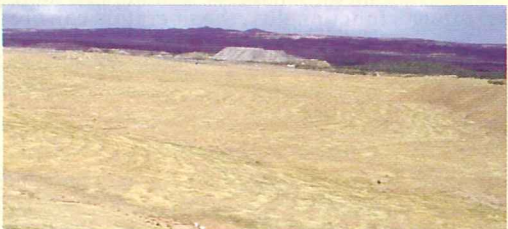
May 5, 2005 – After grading was completed to final design using Dozer 2000-guided equipment, the topdressing was added and seed was applied. Vegetation is beginning to sprout. Note the absence of any rills or gullies despite the landform having endured winter snowmelts and spring rainstorms.
