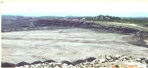
July 10, 2003 – The image is taken from a higher lift against the end-wall looking southeast toward part of the highwall. Precision dumping, guided by global positioning system (GPS), is following the GeoFluv design. The irregular shapes of the outslope piles forming the edges of each lift are visible in the foreground, center right, and upper left. Spot dumping to supplement fill for ridges against the highwall has begun.
