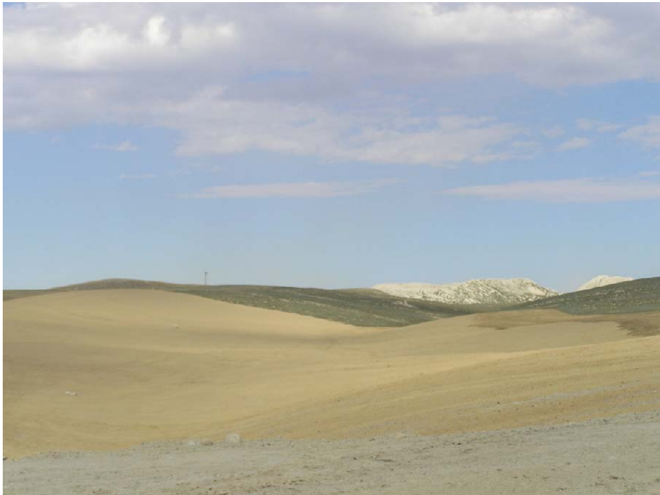
Figure 5. Finished Grading (Fall 2006)
