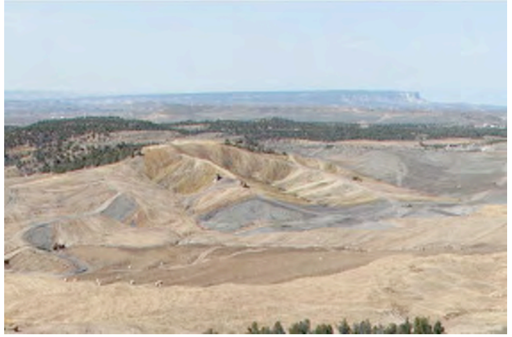
Topdressing lay-down underway at Panel 5 high wall reclamation, Sundance Pit, in 2008
