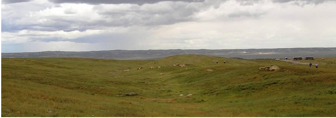
Figure 7. A view of a fluvial geomorphic reclamation area at La Plata Mine that has vegetation starting. The image of a subwatershed headwaters area was captured during the 12 September 2006 National Interactive Forum on Geomorphic Reclamation. The vegetation in the image is just starting and mostly annual plants are visible, representing just the first season's volunteer growth shading the reclamation seeding sprouts.
