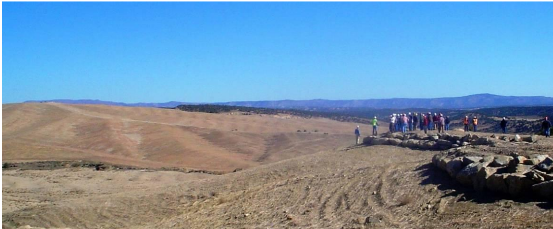
Figure 6. A fluvial geomorphic reclamation area at La Plata Mine that has been topsoiled; all the landform in the fore-ground and mid-ground without tree cover is graded and topsoiled reclamation. Image captured during 28 October 2008 National Association of Abandoned Mine Land Programs national conference tour.
