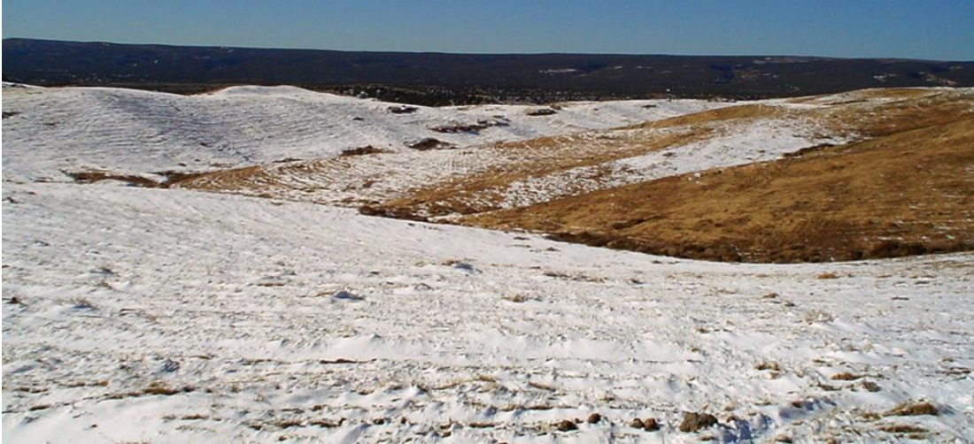
Figure 9. A west-facing view of a constructed GeoFluv™ design that has remained stable after exposure to 25-yr, 50-yr, and 200-yr storm events. The snow covered slopes at the left have a northern aspect and the dominantly south-facing slopes to the right have melted and sublimated their snow cover because of greater exposure to the sun. Note that the subwatershed valleys on the south-facing slope provide additional diversity in moisture harvesting because of their differing exposures to sunlight. In addition to stability against erosion, these slopes provide habitat for diversity in vegetation and wildlife and livestock use.
