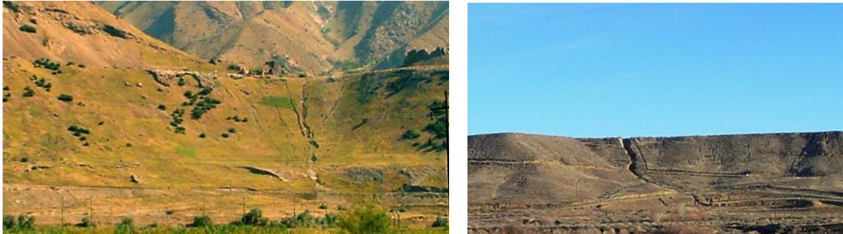
Examples of a water extending channel length on constructed landforms (photograph courtesy of Nicholas Bugosh)
